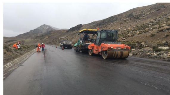
Fig. 5. Paving of WMA at lower compaction temperature
